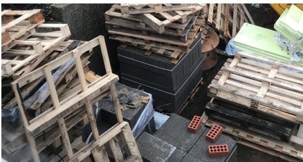
The wooden pallets at Luton site before refurbishment.
